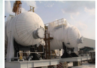
INSULATION MATERIALS TANKS: CALCIUM SILICATE ELLIPTICAL HEAD
