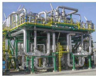
COLD INSULATION C/O GAS COMPRESSION PLANT - STOGIT BRUGHERIO (MI)
