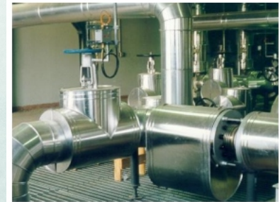
INSULATION MATERIALS TANKS: CALCIUM SILICATE ELLIPTICAL HEAD
